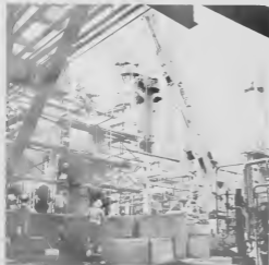
One of the last major jobs the M&C tradesmen had to do on the two feed filters was to load the drums with catalyst.
